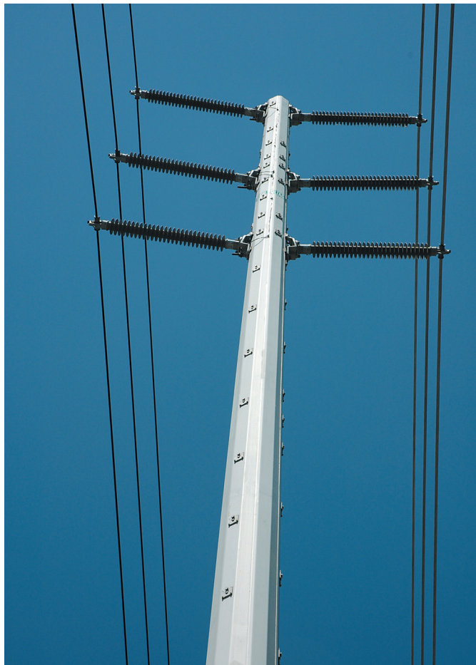
SCE pilot project pultruded transmission pole (left); and at right, modular composite pole for SCE’s “Circuit of the Future”.
