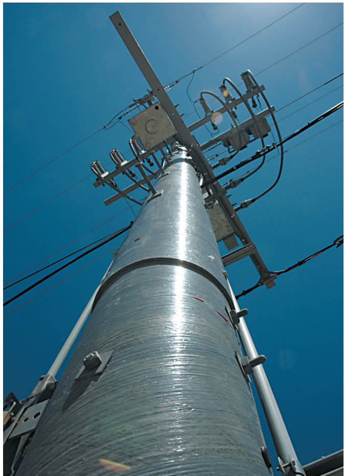
SCE pilot project pultruded transmission pole (left); and at right, modular composite pole for SCE’s “Circuit of the Future”.
