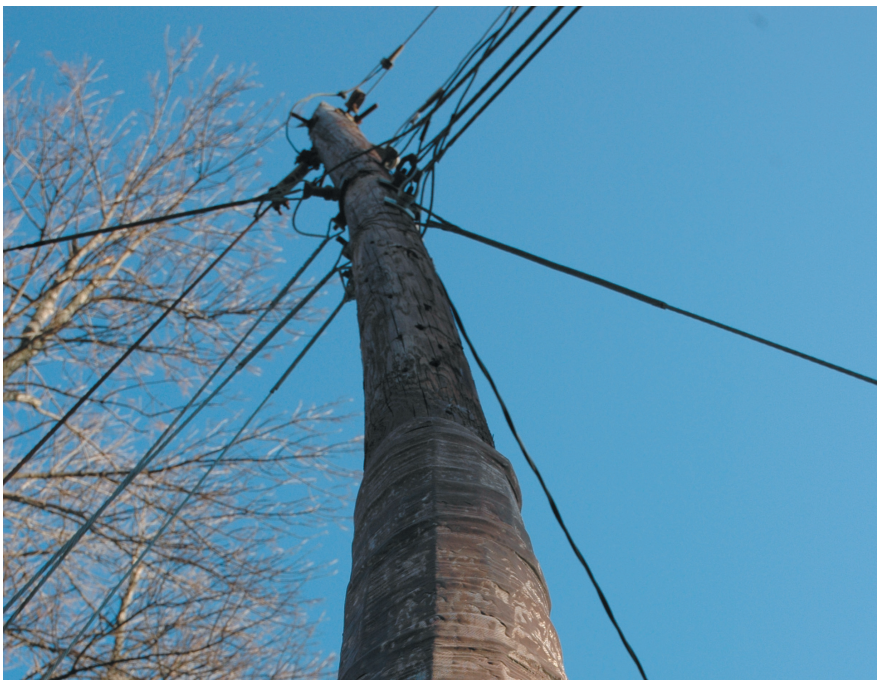
Rapid growth tree farms produce poles that are less robust and do not resist insect infestation or wood rot as well as older generation poles.
