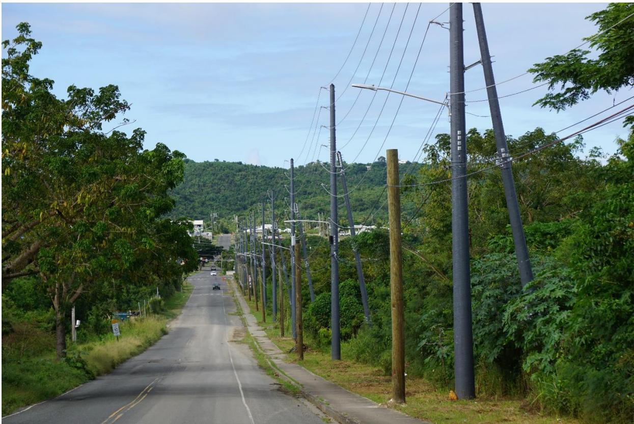
*A line of RS FRP composite utility poles installed in the U.S. Virgin Islands as part of a FEMA hazard mitigation project. These structures are designed to withstand 200mph (320km/h) wind speeds so as to increase system resiliency and harden the electrical grid from the damaging effects of future hurricanes.*
