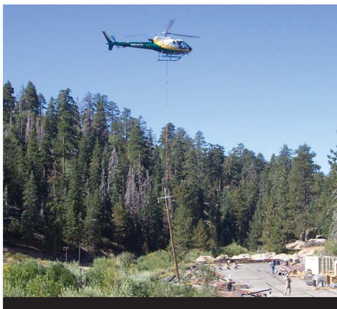
Even fully assembled, the composite pole is substantially lighter than wood or other materials and easily transported by a helicopter.
