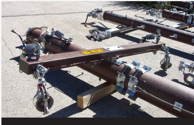
These composite poles are framed with composite crossarms ready for helicopter transport to the mountainous installation location.
