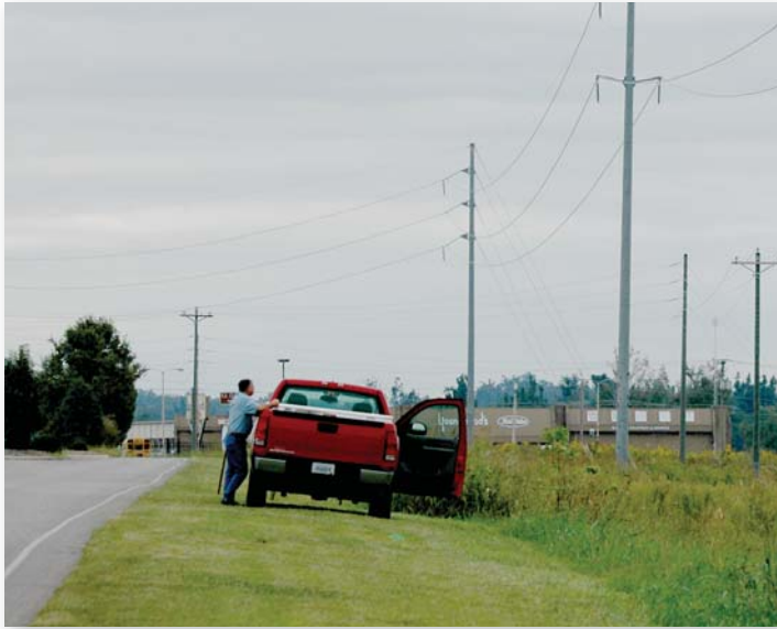
This distribution line was constructed with composite poles alongside, and the transmission line was constructed with steel poles.
