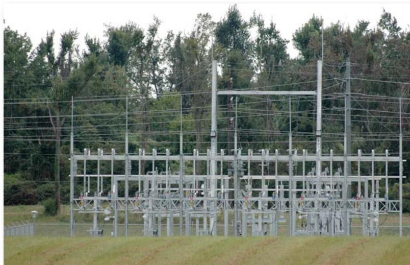
A composite pole was used for a 69-kV transmission switch pole connection into a new distribution substation.
